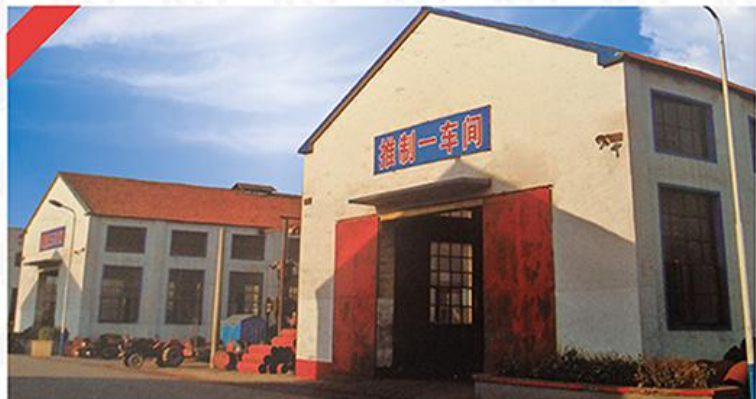
推制一, 三车间 NO. 1 AND 3 EXTRUDING WORKSHOP
